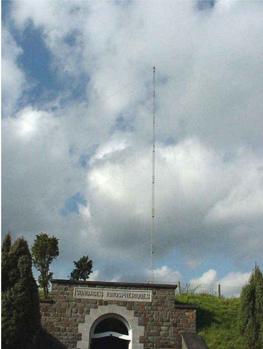
**Fig. 65.3e.** The entrance of the digisonde station at Dourbes. The 42-meter supporting mast for the vertically pointing asymmetrical rhombic transmitting antenna is clearly seen on top of the digisonde station.
